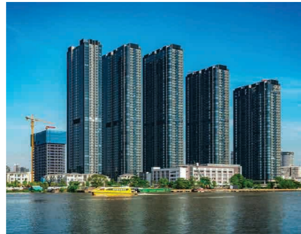
Install stainless steel pipes for Vinhomes Bason
